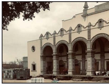
GWS Auditorium façade. New front steps are part of the construction.
