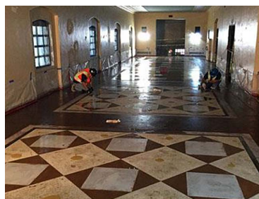
2nd floor terrazzo installation
