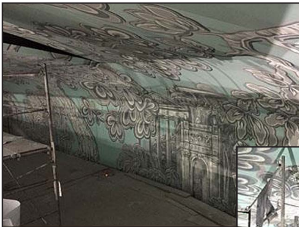
Mural with scaffolding in place
